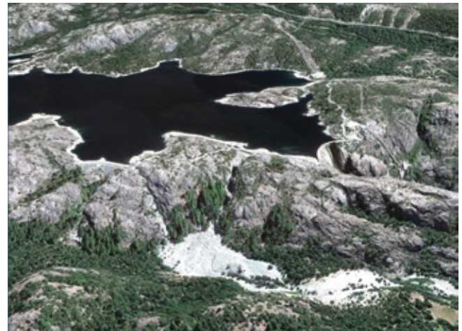
2 | Google Earth view of Spaulding Lake Dam where dam erodibility research was conducted.
