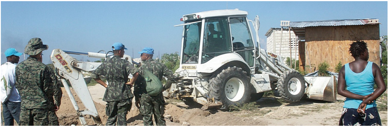
3 | Digging of new water well in Onaville with collaboration of UN-MINUSTAH, UNASUR and TECHO
